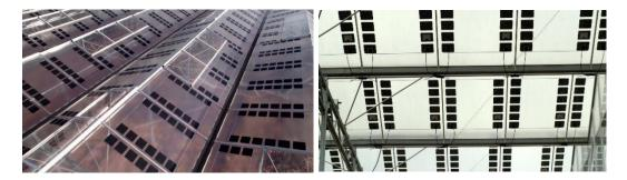
Figures 6,7: Brite Solar Glass Panel designed for vineyard greenhouse cultivation.
