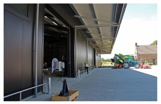
Figure 3: Front view of the "Bewaarschuur van de Toekomst" with wide crossing of the rooftop, creating a lot of shadow on the walls and around the building.
