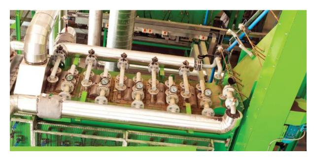
Figure 5: Derived hot flue gas (at  $> 850^{\circ}$ C) travels through a number of heat exchanger flue gas to hot water (or steam) tubes.
