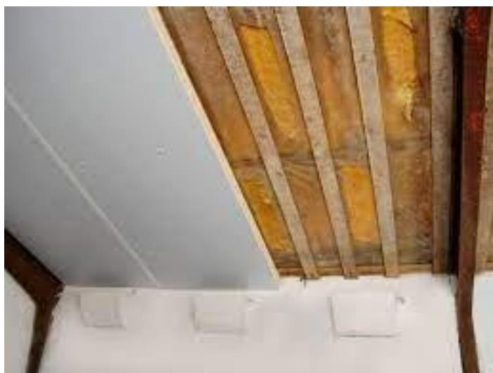
**Figure 1:** Ceiling insulation of old pig stable using polyisocyanurate (PIR) (source: Recticel Insulation)
