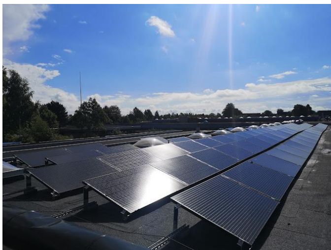
Figure 1: Solet solar panel system set up on a roof
