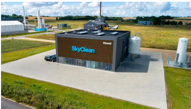
Figure 1: Fully automated 2 MW plant located in GreenLab near Skive, Denmark (Photo, Stiesdal)
